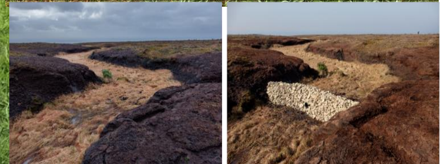
Headwater drainage 'Stone dams', Stalybridge, 3,000 m3 vol,
